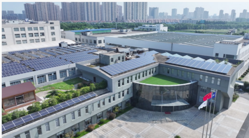
Roof Photovoltaic of Wuxi Manufacturing Base, Jiangsu
