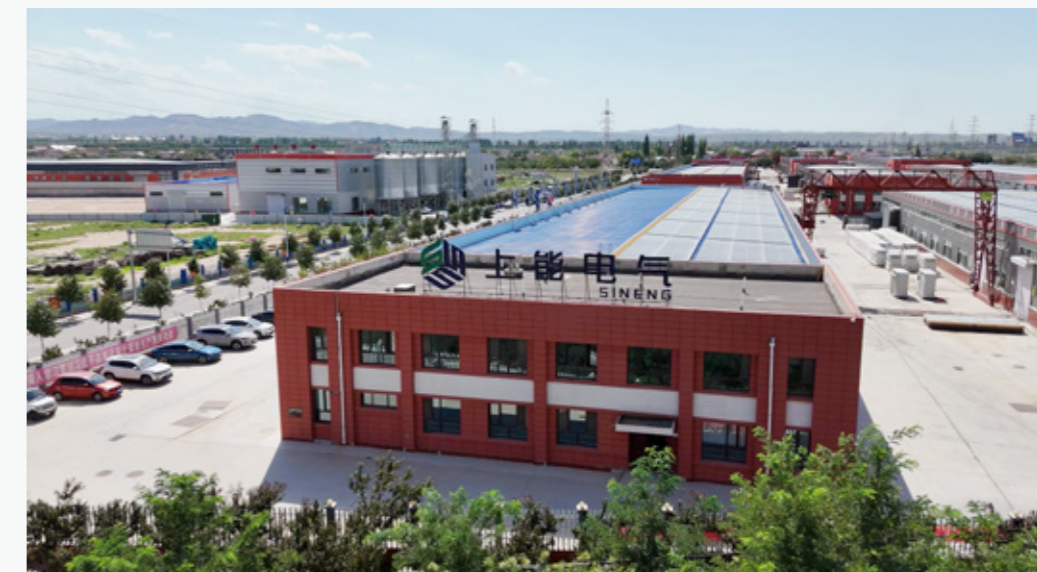
Roof Photovoltaic of Wuzhong Manufacturing Base, Ningxia
